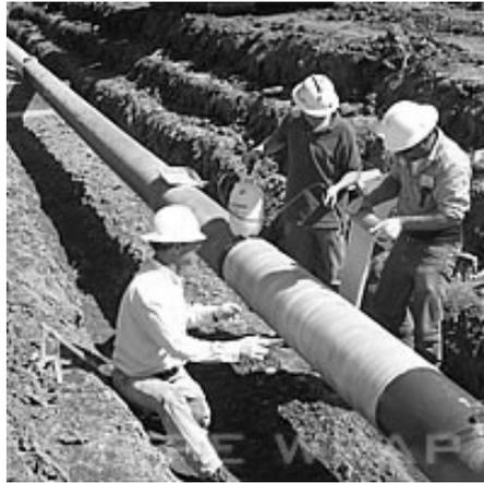
**Figure 1: Repairing process of a damaged gas pipeline by wrapping of impregnated fiber fabric over the defected area [4]**
