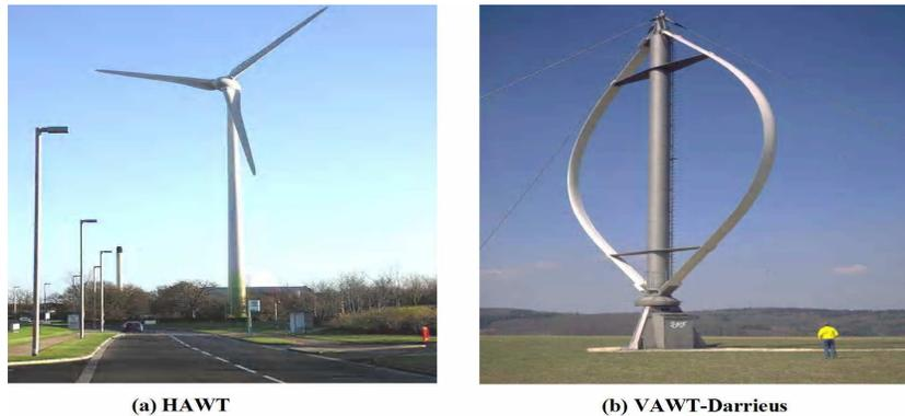
**Figure 1: Basic Types of Wind Turbines**
