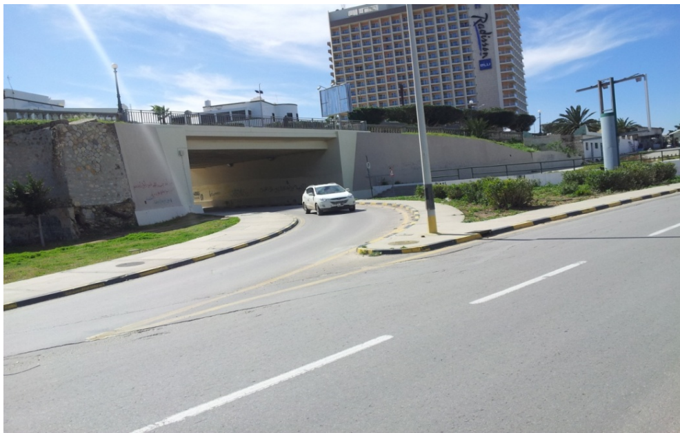
Figure 3: A side view of Al Mahary Bridge
