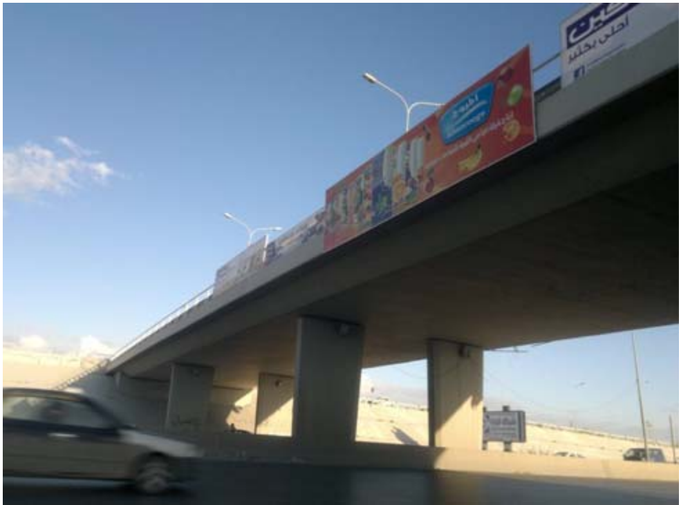
Figure 2: A lower side view of Al Khazanat Bridge
